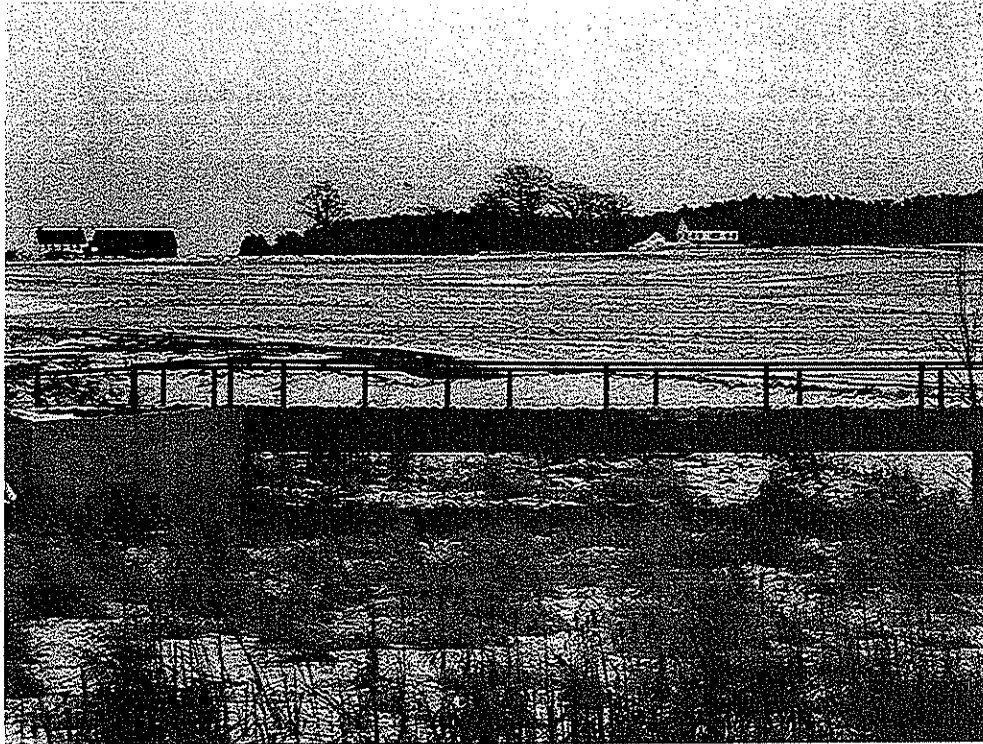
Lewis Family Farm bridge over wetlands with farm office, farm barn, and farm manager's house in background.
